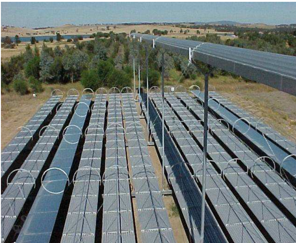
Fig.3: Image of a CLFR collector commissioned in Australia by Solar Heat and Power Pty. Ltd.
